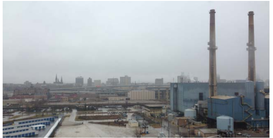
all images taken with verbal permission from Elevator E site visit - 12-21-2015
