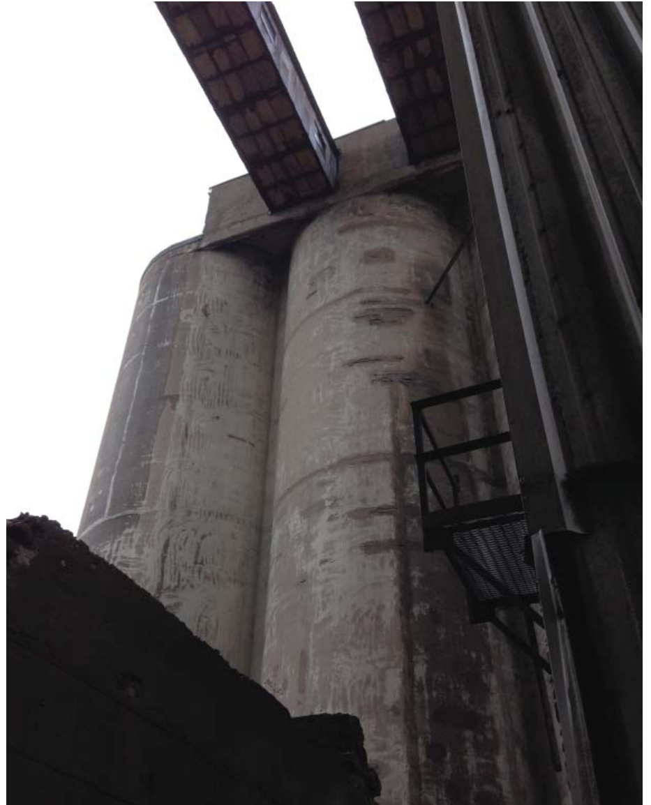
all images taken with verbal permission from Elevator E site visit - 12-21-2015
